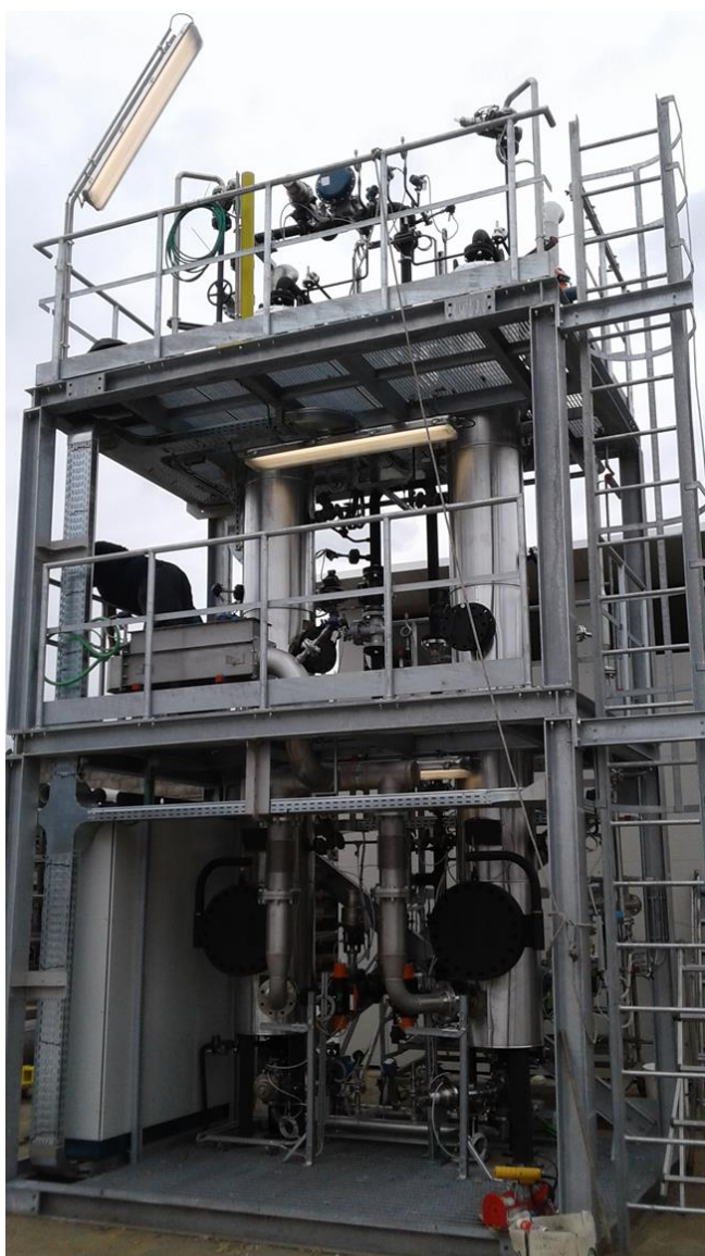
Figure 1: Pilot plant during construction operations
