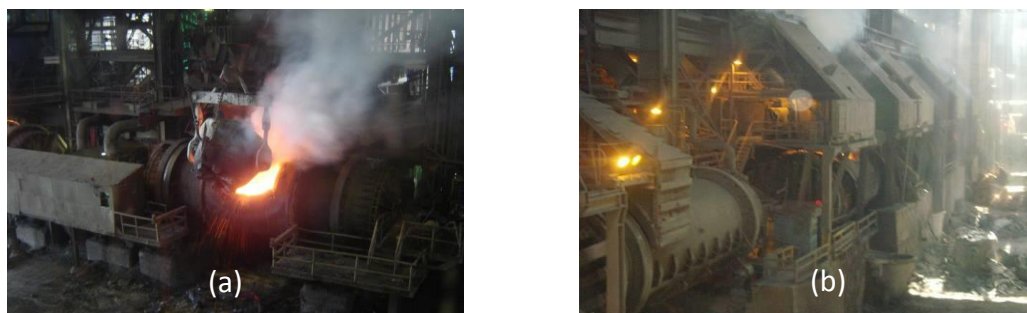
Figure 1: Fugitive gases from the matte charging of conversion process (a) and CPS converters equipped with secondary hood (b).
