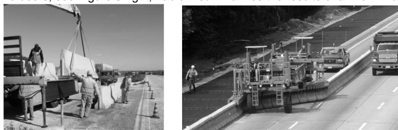
Figure 3: Barrier transfer: traditional procedure (left), mechanized “Barrier Zipper” technique (right).
