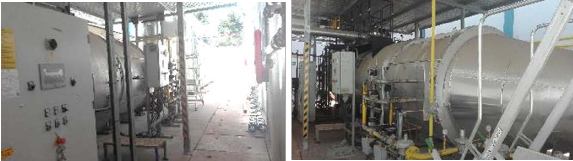
Figure 1: Cogeneration plant (CHP) serving the pasta factory studied: microturbine (left), after-burner (right)
