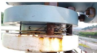
Figure 2: Damaged spiral.
