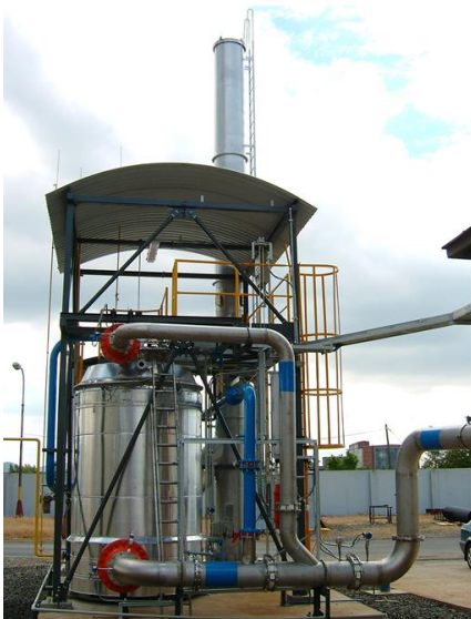
Figure 4: Industrial application of compact MIE technology for waste gas thermal treatment.
