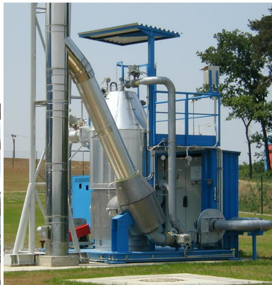
Figure 4: Industrial application of compact MIE technology for waste gas thermal treatment.
