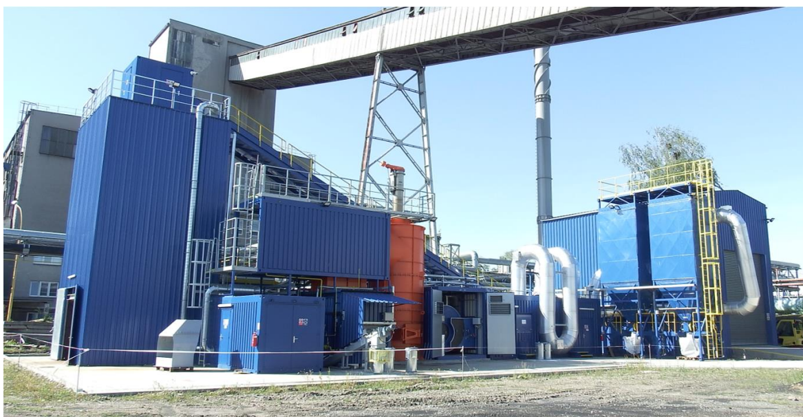
Figure 2: EVECONT – micro incineration unit for thermal processing of plastic non-recyclable waste
