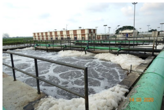
Figure 3: MBBR technology implemented in WWTP of Soekarno-Hatta Airport
