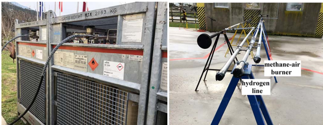
Figure 1: Storage facility (left) and hydrogen release line and methane-air burner (right).
