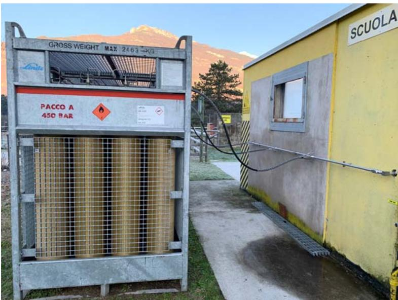
Figure 2: The storage tube trailer supplied by Linde.
