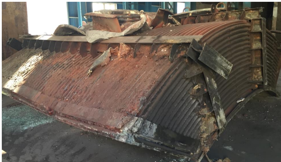
Figure 3: Broken hood from the smelting plant
