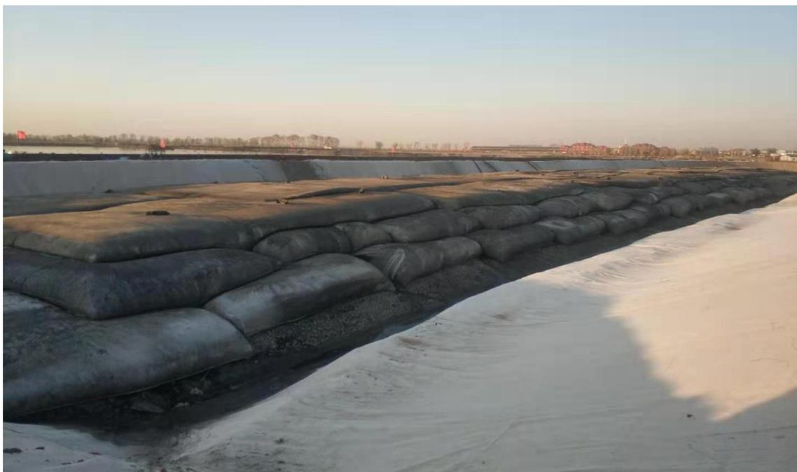
Figure 5: Dewatering in geotextile tubes
