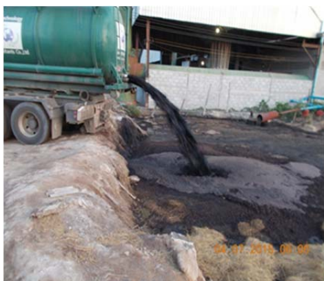
Figure 1: The sludge from wastewater treatment system.
