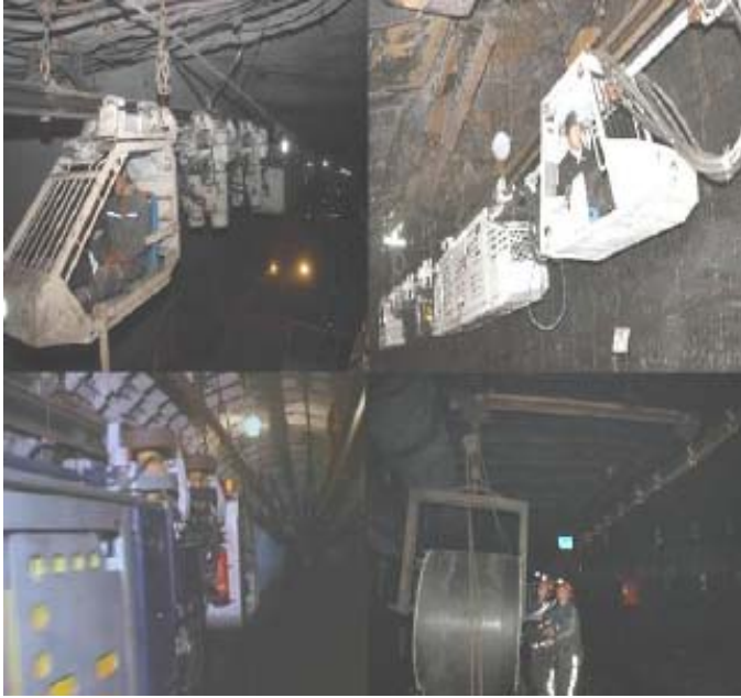
Figure 2: The Tunnel in Coal Chemical
