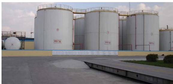
Figure 1: chemical storage tank farm
