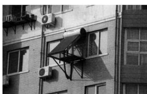
Figure 2: Installation of solar water heater on an elevation Figure 3: Installation of solar water heater on the wall between windows and window-sill wall
