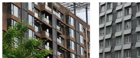
Figure 2: Installation of solar water heater on an elevation Figure 3: Installation of solar water heater on the wall between windows and window-sill wall
