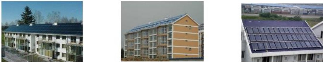
a) Wall-to-wall arrangement of collector b) Local arrangement c) Arrangement of vacuum tube type collector
