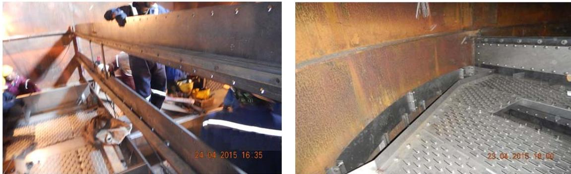
Figure 5a: Installation of the Dividing Wall in the FCC Naphtha Splitter at an Indian Refinery; Figure 5b: Dividing Wall Internals inside the Tower
