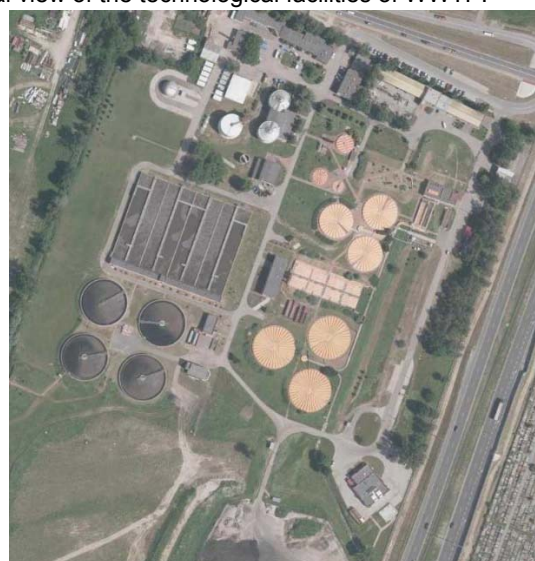
Figure 2 The location of the technological facilities of WWTP (before modernization and extension)
