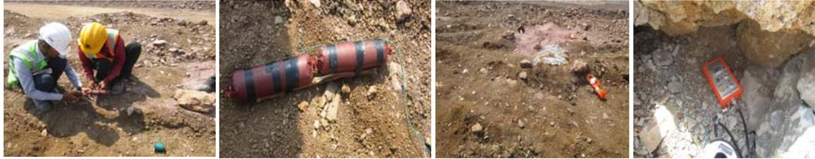
Figure 2: Snapshot of VOD measurement using Handitrap-II.
