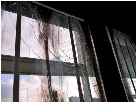
Figure 5: First glass of the triple-pan window
