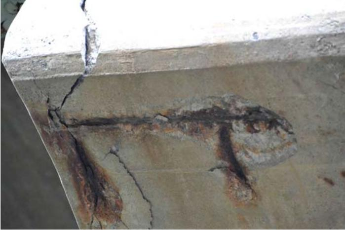
Figure 1: Reinforced concrete damaged by sulfate erosion
