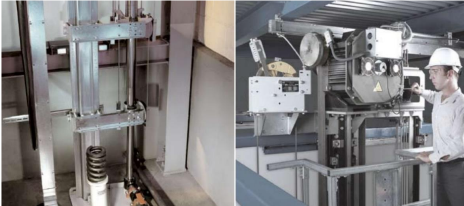
Figure 1: Eco-friendly elevators that utilising telescoping jack systems (left); Machine room-less (MRL) elevators (right) (Schindler, 2017)
