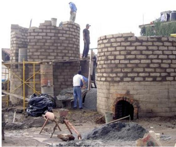
Figure 1: Construction of new brick kilns
