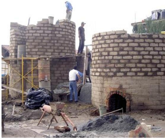
Figure 1: Construction of new brick kilns
