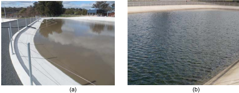
Figure 1: Near-smooth (a) and wavy conditions (b) for liquid surfaces in an WWTP.
