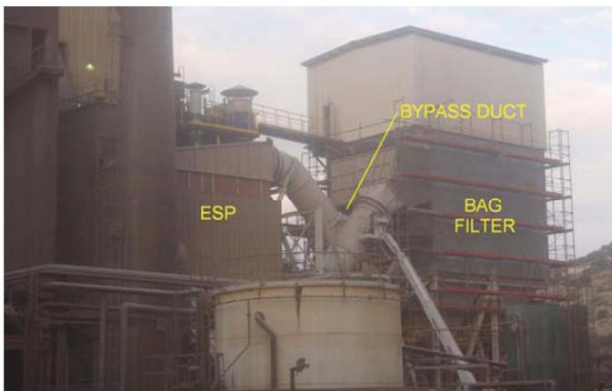
Figure 1: Example of a hybrid dedusting system constituted by an ESP coupled with a bag filter.
