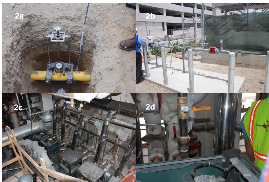
Figure 2: Gas delivery: incoming line (2a), meter set assembly (2b), 5 th floor fuel manifold (2c), and water boiler feed (2d)
