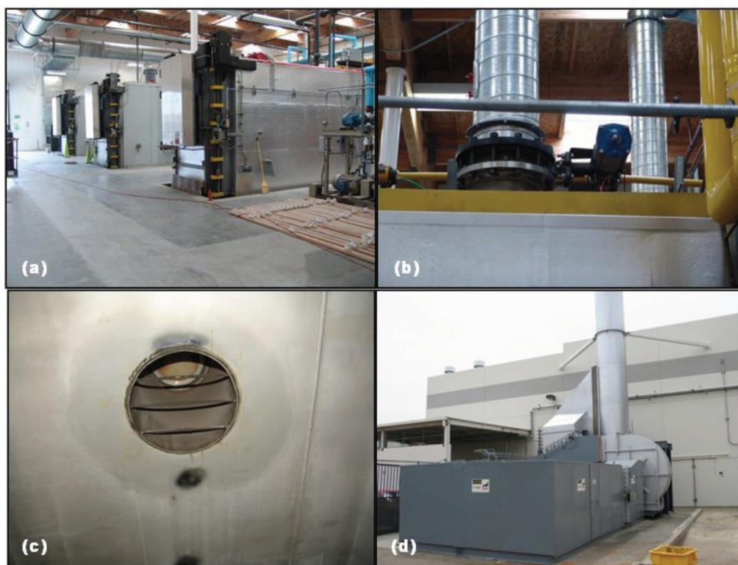
Figure 2: Sterilization chambers after facility reconstruction (a), backvent valve and duct (b), interior view of backvent (c) and catalytic oxidizer (d).
