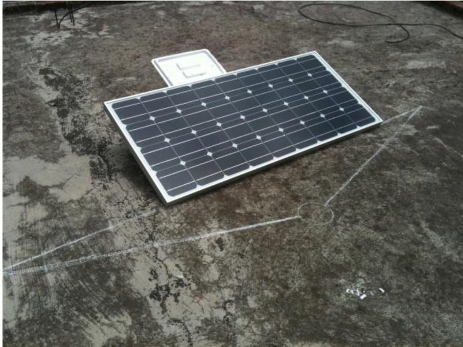
Figure 3: Mono-crystalline Solar Panel.
