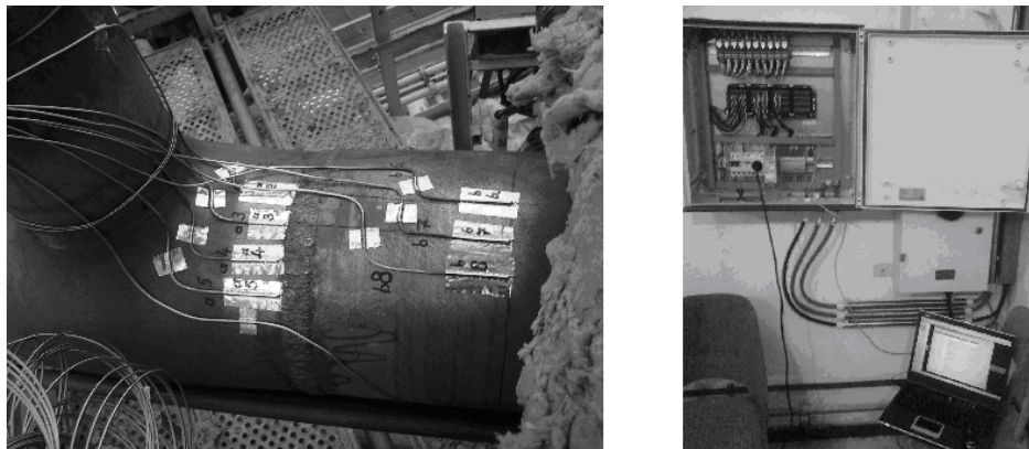
Figure 5 Measurements performed at the hydrocrack nozzles
