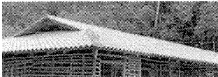
Figure 11. Roof with clay tiles
