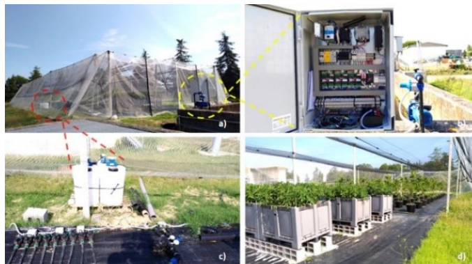
Figure 1. "Smart" pilot system.
