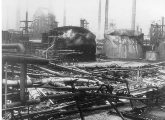
Fig.1: Vapour cloud explosion debris in a refinery in 1968.
