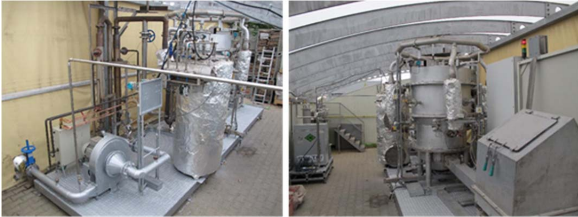
Figure 1: Autothermal gasification technology: a) gas cleaning devices - hot filter, gas cooling and exhaust fan; b) fuel bin and fuel transport into autothermal gasifier.
