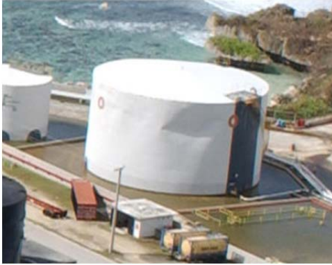
Figure 2: Buckling of a tank in the island of Guam, under a hurricane, 2002 (LEF - Learning from Engineering Failures, s.f.).
