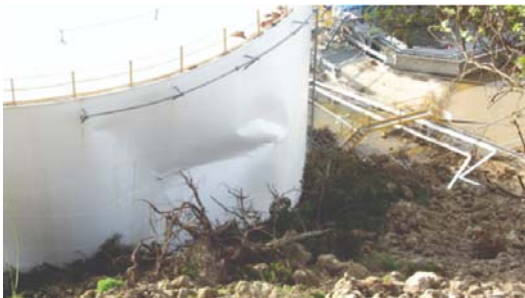
Figure 4: Storage tank damaged by landslide debris, 2014 (GNS Science, 2014).
