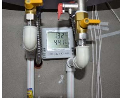
Figure 8: The temperature and humidity recorder between the water storage tank and the hole
