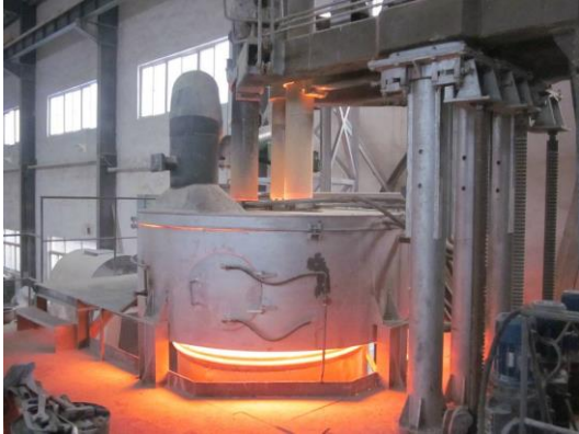
Figure 1: Intelligent control of electric melting furnace
