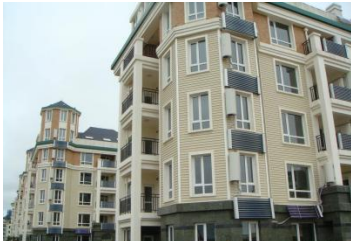
Figure 3: A wall-mounted solar water heater
