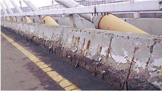
Figure 1: An example of sulfate corrosion
