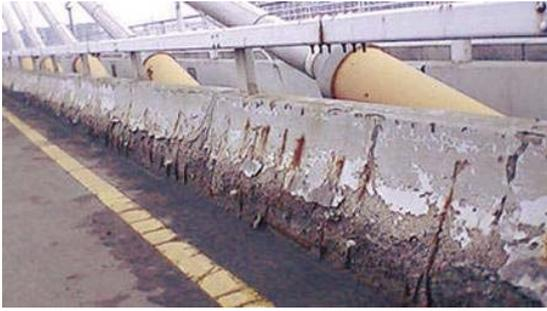
Figure 1: An example of sulfate corrosion
