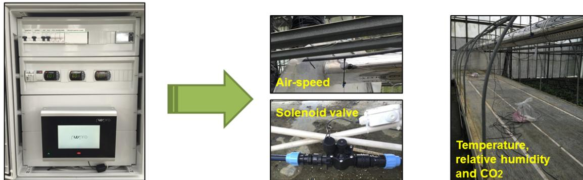
Figure 2: Control panel with a I/O module, 3 parametric controllers and an energy meter
