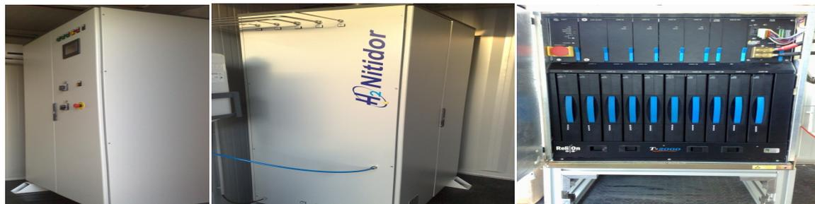
Figure 2: Control system, electrolyzer internal stack and fuel cell of the stand-alone hydrogen plant.
