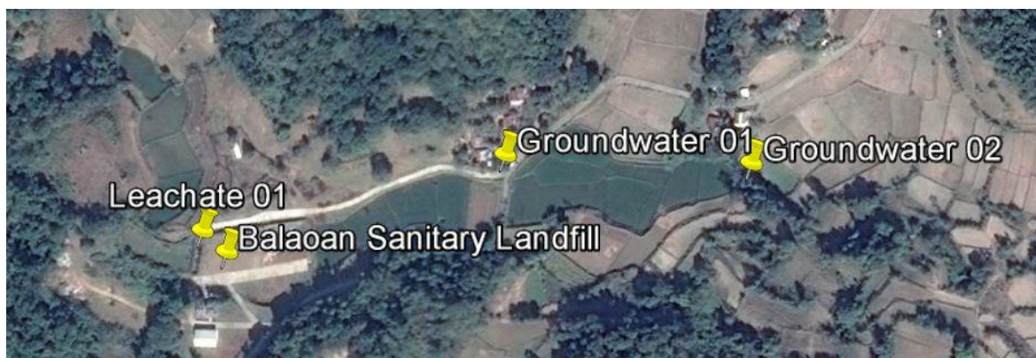
Figure 1: A view of the sanitary landfill showing the groundwater sampling sites.
