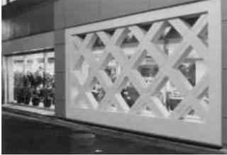
Figure 1 (a): grid shear wall
