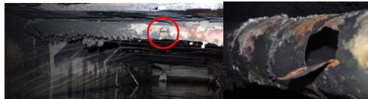
Figure 4: Photos of the storm water trench, the 4-in propylene pipeline and the break.
