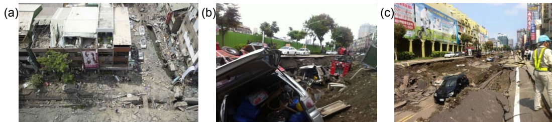
Figure 2: Photos showing the explosion damage near (a) the junction of Sanduo 1 st road and Wuqing 2 nd (b) the south side of Kaixuan 3 rd road and (c) Yixin 1 st .
