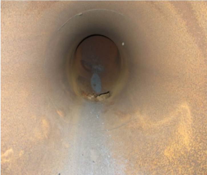
Figure 3: View in the main pressurized air pipeline
