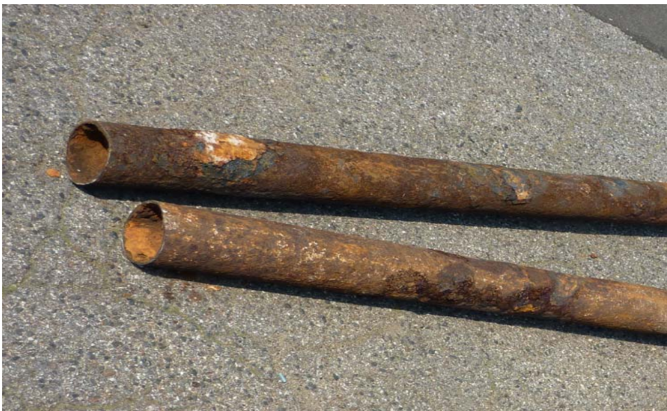
Figure 2: Samples of downstream cooling water pipelines in the production building showing significant corrosion and reduction of wall thickness.
