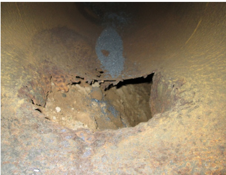
Figure 4: Detail view on the corroded area
