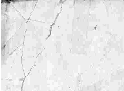
Figure 1: Tree crack
