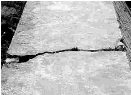
Figure 2: Horizontal crack
