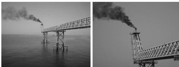
Figure 2: Black smoke in flare of phase 1 platform
