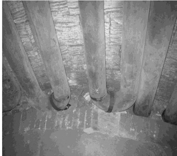
Figure 2: Important geometry imperfection in the bottom part of radiant coil
