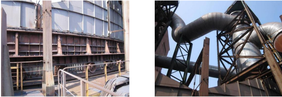
Figure 1: A sinter cooling bed of Anshan Steel (a) Trolley, (b) Hoods
