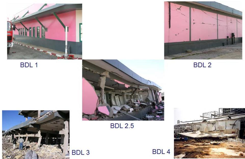
Figure 2. Building Damage Level Categories (Examples)
