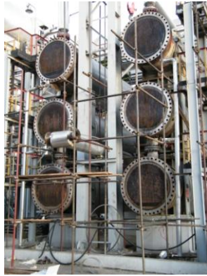
Figure 9: 6 shell exchanger; 30,000 tubes, partial condensation on the tubeside. (Courtesy of Lukoil, Russia)
