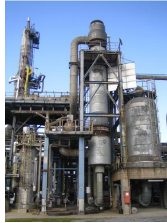
Figure 8: Texas Tower (Courtesy of Ruhr Oel, Gelsenkirchen, Germany)
