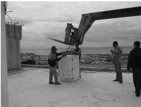
Fig 4: Fuel Cell installation and front view of the site.
